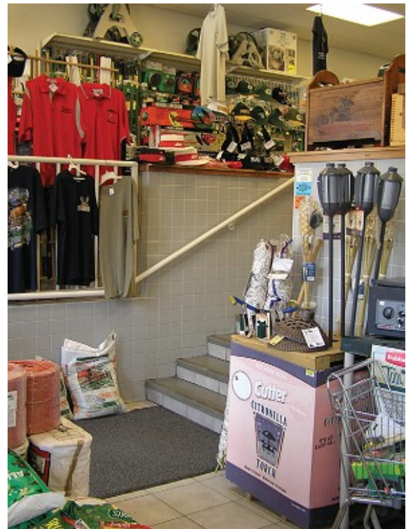
After entering the business, shoppers can either go up the ADA compliant ramp (left) or go up the stairs to the new first floor level (right). The entrance area has been retrofitted with flood resistant materials including a tile floor and tile surfaces on the stairs (Darlington, Wisconsin, photos courtesy of FEMA).
