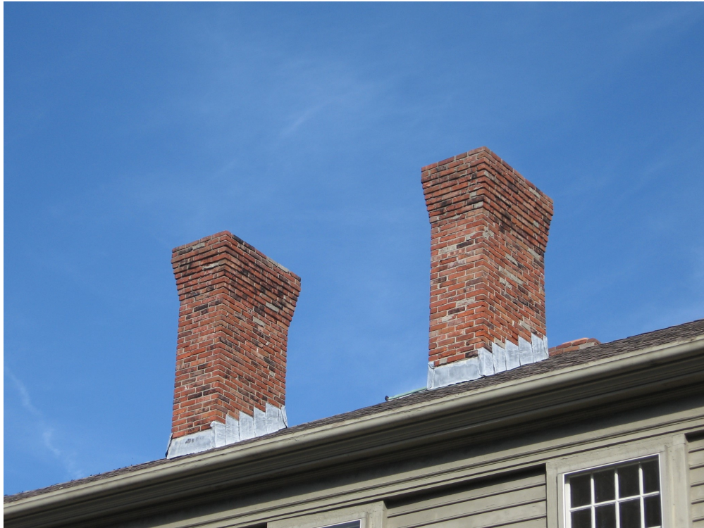
Most chimneys in the Newport Historic District are of brick and are located on the interior rather than on exterior walls. In an elevation project these chimneys should be elevated along with the rest of the house and kept at their original locations (above, 59 Bridge Street and below, 54 Thames Street).
