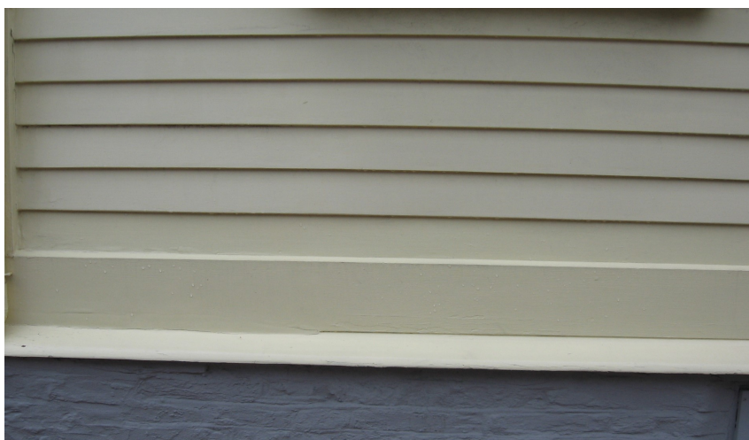
The dwelling at 14 Third Street displays a wide skirt board which would be appropriate for an elevation project.
