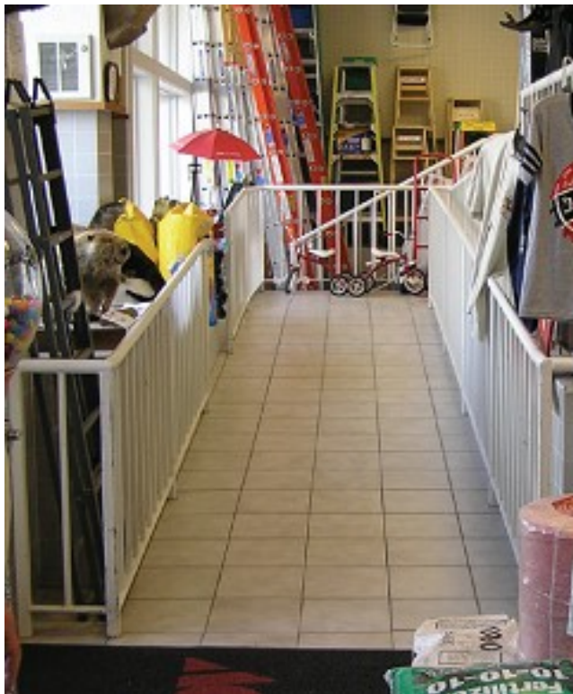
After entering the business, shoppers can either go up the ADA compliant ramp (left) or go up the stairs to the new first floor level (right). The entrance area has been retrofitted with flood resistant materials including a tile floor and tile surfaces on the stairs (Darlington, Wisconsin, photos courtesy of FEMA).
