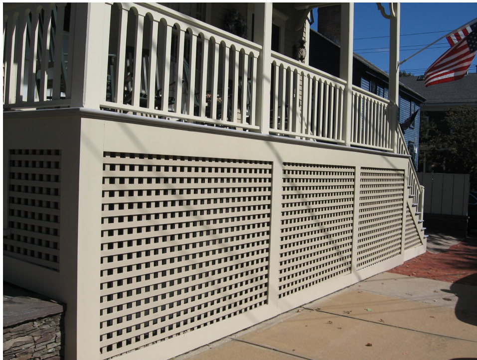
The dwelling at 27 Walnut Street displays recessed lattice panels in traditional square designs and these types of panels are appropriate for porches in elevation projects.
