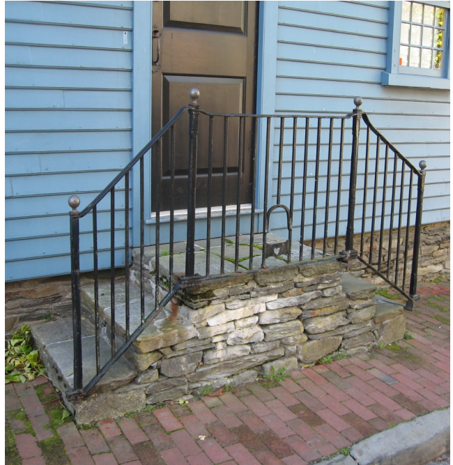
Appropriate stair designs for elevated buildings include the side/linear stair of brick construction at 11 Third Street (left) and the center/linear split wood stair of stone at 6 Bridge Street (right). Both have iron posts and railings in traditional Newport designs.
