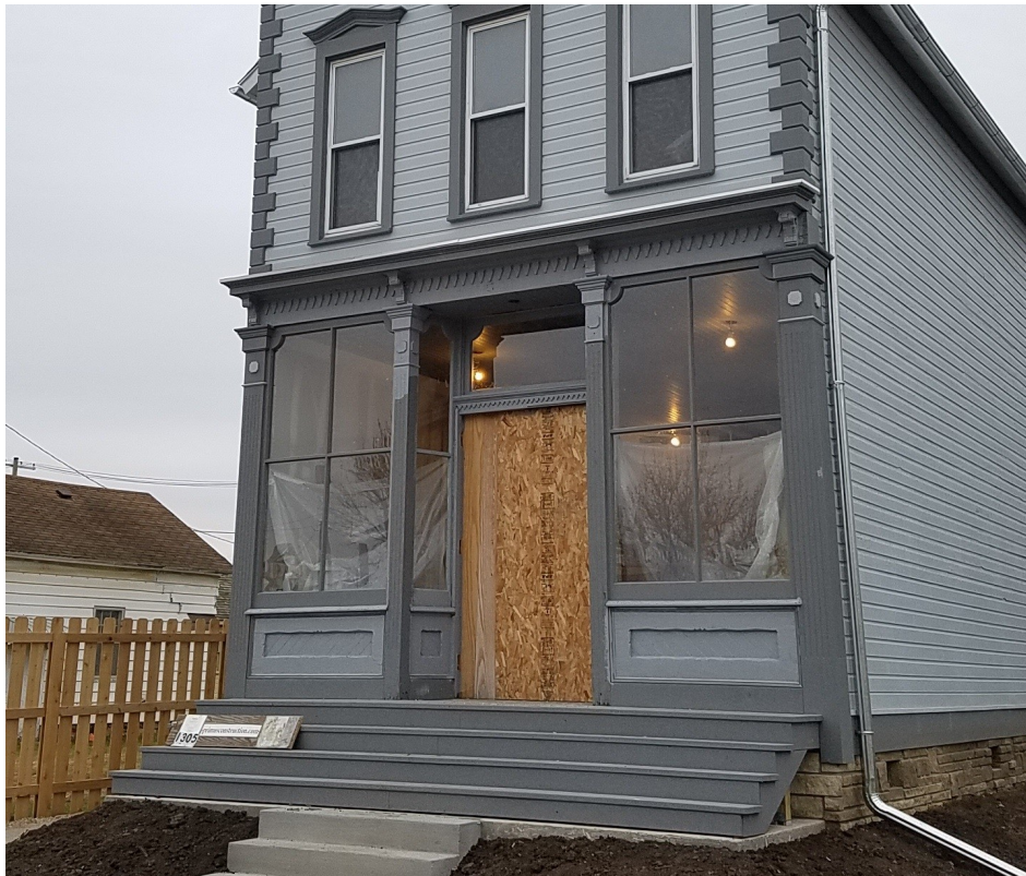
Commercial buildings in the Newport Historic District which may require elevation include 27 Second Street (above). The commercial building shown below was elevated by increasing the grade height, adding a new brick foundation and new stairs. An ADA compliant ramp and entrance was added at the rear (Cedar Rapids, Iowa, courtesy of Chris Wand).
