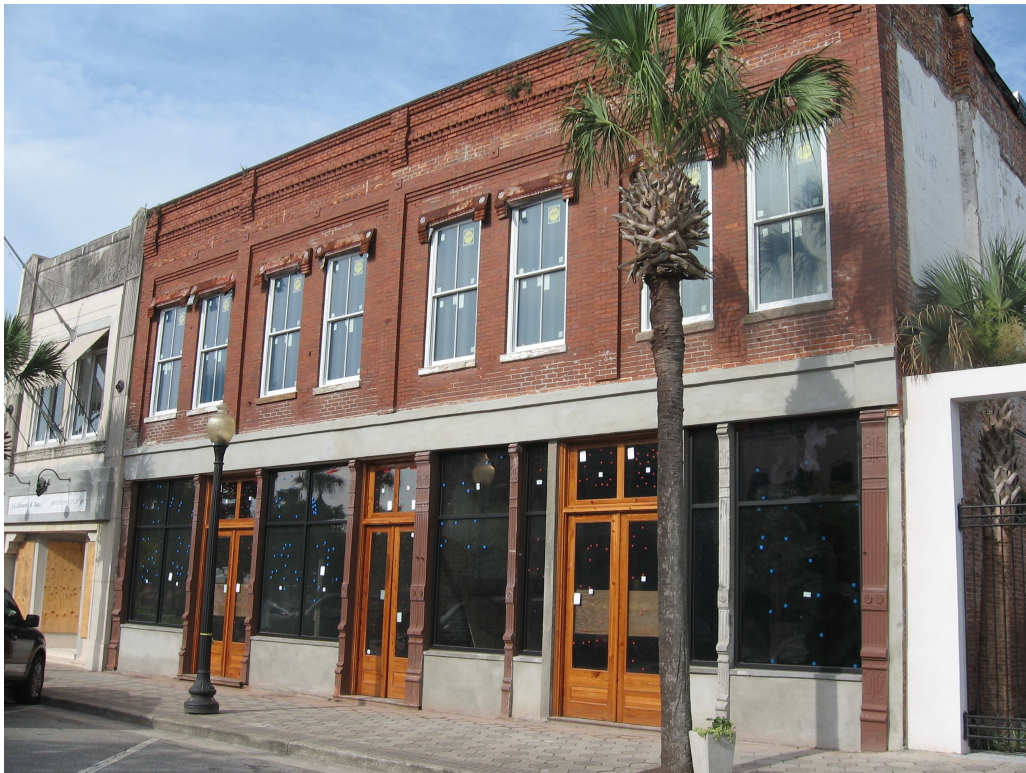
The rehabilitation of this historic commercial building included the hardening of the bulkheads (the panels beneath the display windows) through the replacement of the wood panels with concrete and a parged surface to withstand flooding (Brunswick, Georgia).
