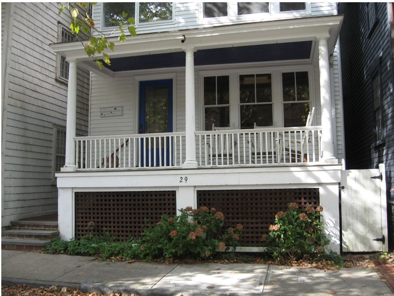
The dwelling at 29 Willow Street displays common porch elements to be retained in an elevation project such as porch column and foundation pier alignment, appropriate lattice panels and a wide skirt wall between the porch and foundation.
