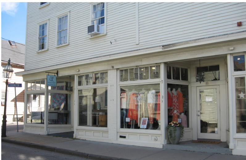
The commercial building at 78-80 Thames Street has frame bulkheads which could be protected by flood shield panels.
