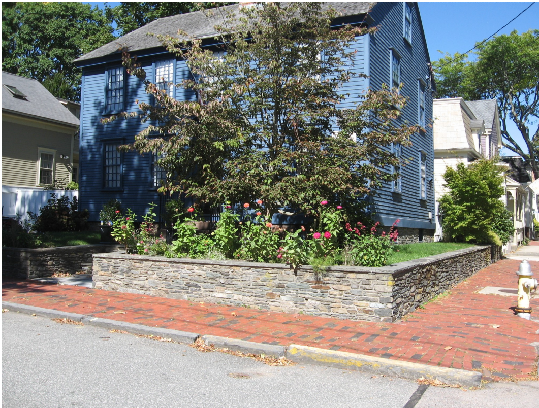
At some time after 1950, this dwelling was elevated and moved back on its lot. The property was then placed on a higher grade and landscaped with a stone retaining wall. This approach is recommended where the lot size allows the house to be moved back from the street.
