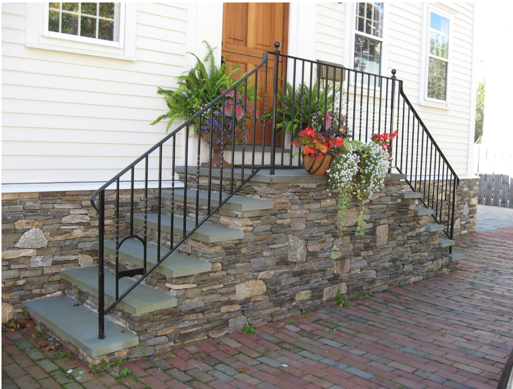
Past elevation projects in the Newport Historic District include those at 74 Bridge Street (above) and 62 Bridge Street (below). In both cases, new center/linear split stairs were added with materials to match the foundation and appropriate iron railings.
