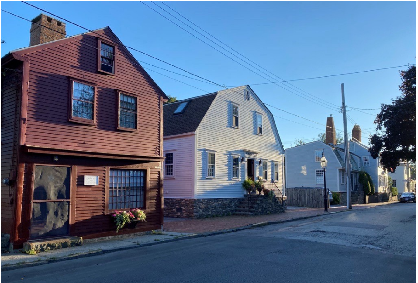
Bridge Street in Newport offers examples of buildings elevated and set back beside neighbors on grade.
