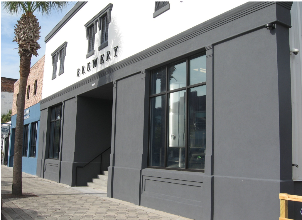
New commercial buildings in the flood zones should be designed with hardened storefronts such as the concrete bulkheads and elevated first floors on these buildings. ADA compliant entrances are located on side elevations (Brunswick, Georgia).
