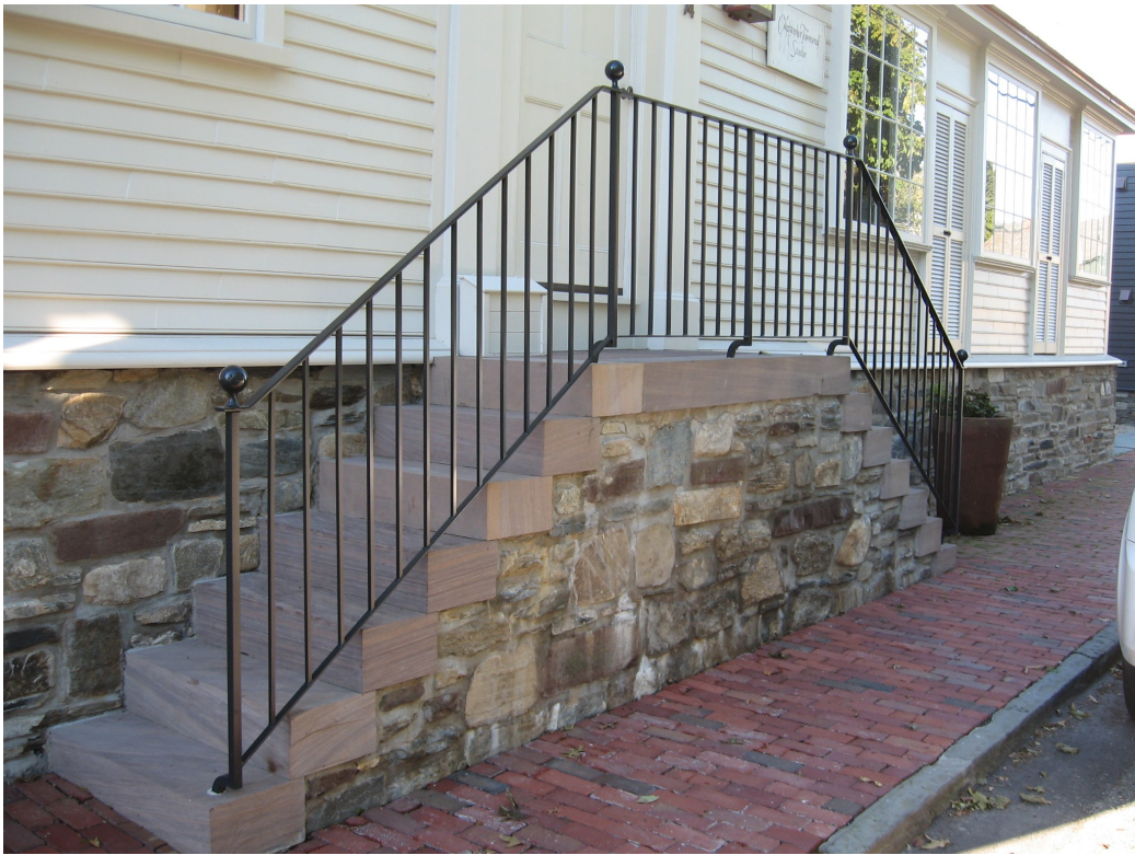
Past elevation projects in the Newport Historic District include those at 74 Bridge Street (above) and 62 Bridge Street (below). In both cases, new center/linear split stairs were added with materials to match the foundation and appropriate iron railings.
