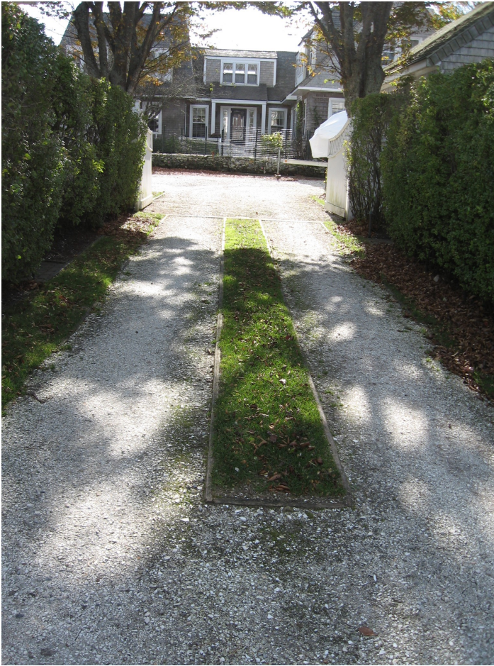
YES: Property owners are encouraged to use permeable materials for driveways such as gravel instead of hard surfaces like concrete or asphalt (left). Another approach is to only hard surface the driveway “ribbons” as shown at right (Nantucket, Massachusetts).
