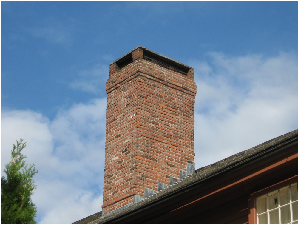
Most chimneys in the Newport Historic District are of brick and are located on the interior rather than on exterior walls. In an elevation project these chimneys should be elevated along with the rest of the house and kept at their original locations (above, 59 Bridge Street and below, 54 Thames Street).
