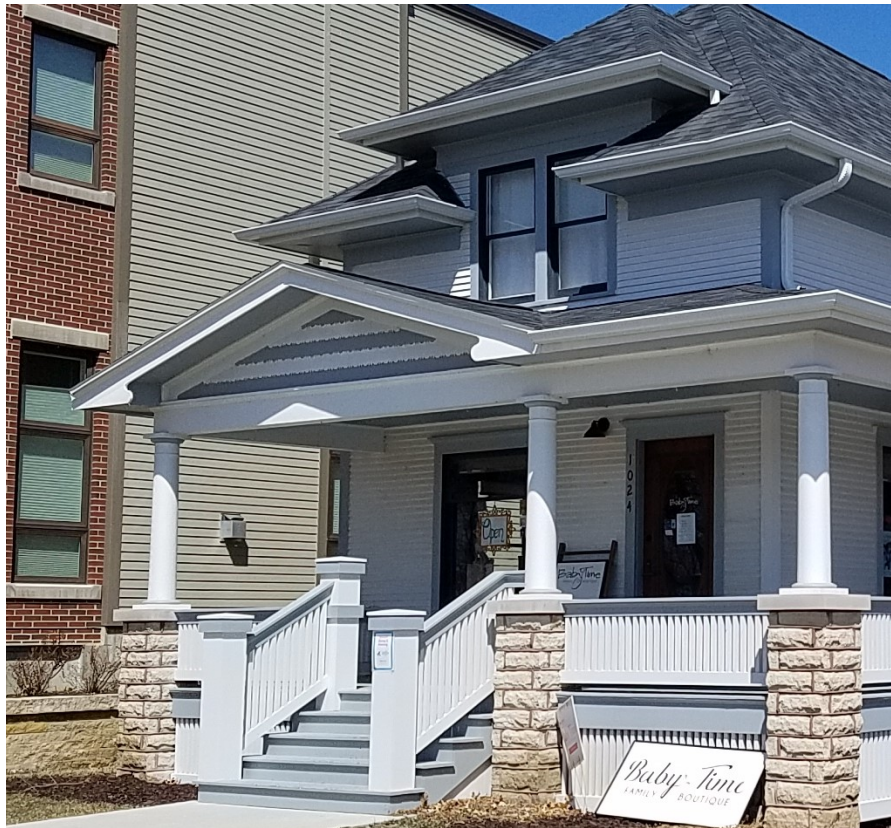
The porch piers on this elevated dwelling were increased in height using stone salvaged when the foundation was rebuilt (Cedar Rapids, Iowa, photo courtesy Chris Wand).
