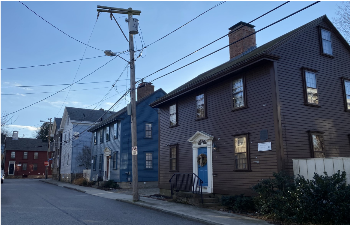
Dwellings on most blocks in the Newport Historic District are consistent in their height, setback, street orientation, and materials.
