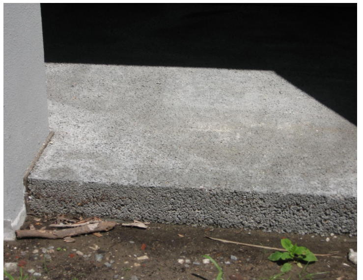
YES: Permeable pavement materials should also be considered for new or replacement parking areas to limit water runoff and ponding (Charleston, South Carolina).
