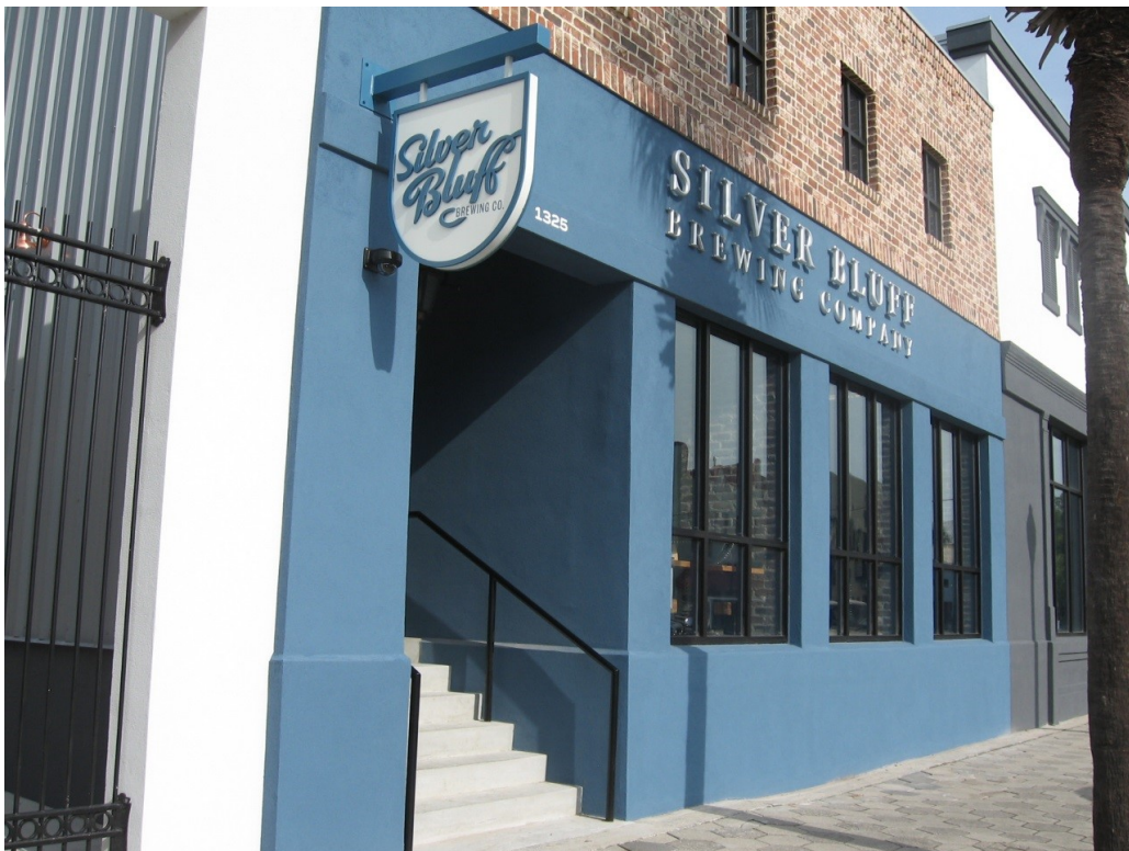
New commercial buildings in the flood zones should be designed with hardened storefronts such as the concrete bulkheads and elevated first floors on these buildings. ADA compliant entrances are located on side elevations (Brunswick, Georgia).
