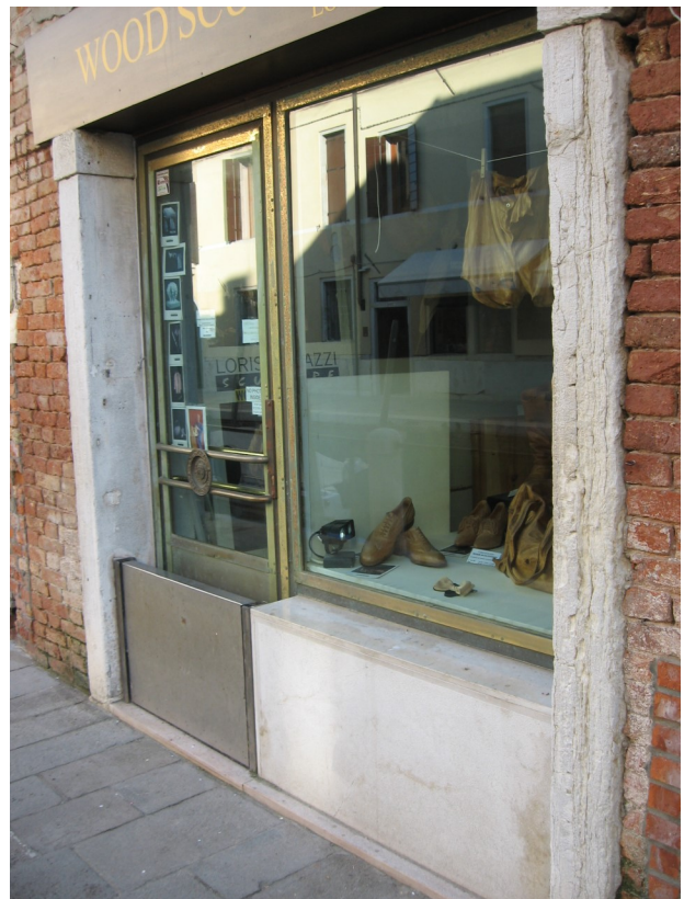
Examples of flood shields to protect entrances. The photo above shows a shield and shield track in deployed position (Venice, Italy).
