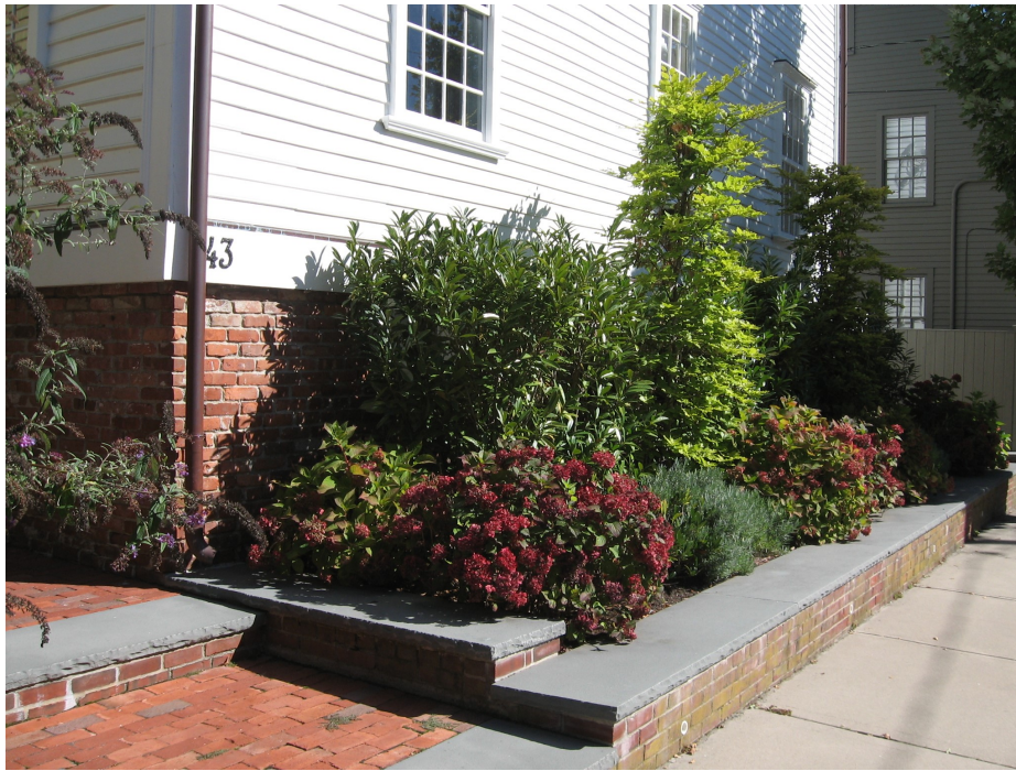
The dwelling at 43 Elm Street illustrates how low planter walls and landscaping can reduce the visual effects of foundation height.
