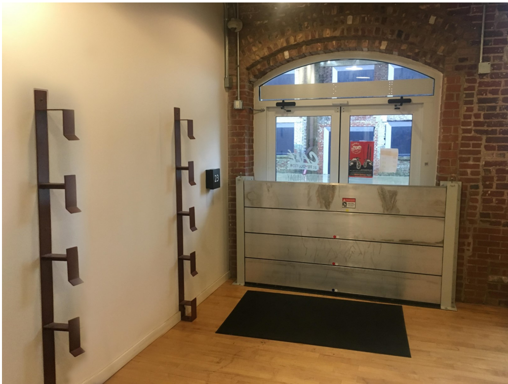
Flood shields for commercial buildings can be stored in the building as shown above and then deployed to protect the building during periods of high water (below) (New Bern, North Carolina, courtesy of the North Carolina State Historic Preservation Office).
