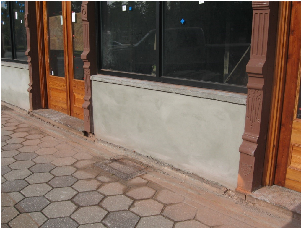
The rehabilitation of this historic commercial building included the hardening of the bulkheads (the panels beneath the display windows) through the replacement of the wood panels with concrete and a parged surface to withstand flooding (Brunswick, Georgia).
