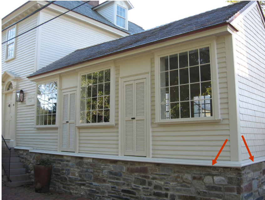
The elevation of 74 Bridge Street included the addition of a wide water table between the foundation and wood siding.
