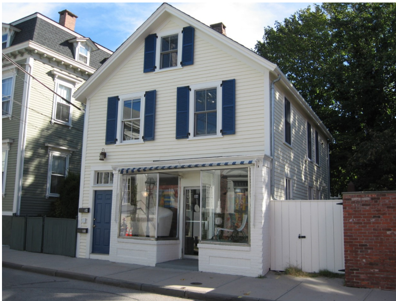
The commercial building at 86 Thames Street retains original brick bulkheads at the storefront which provides some flood resistance. Flood shields could be deployed to protect the entrances.
