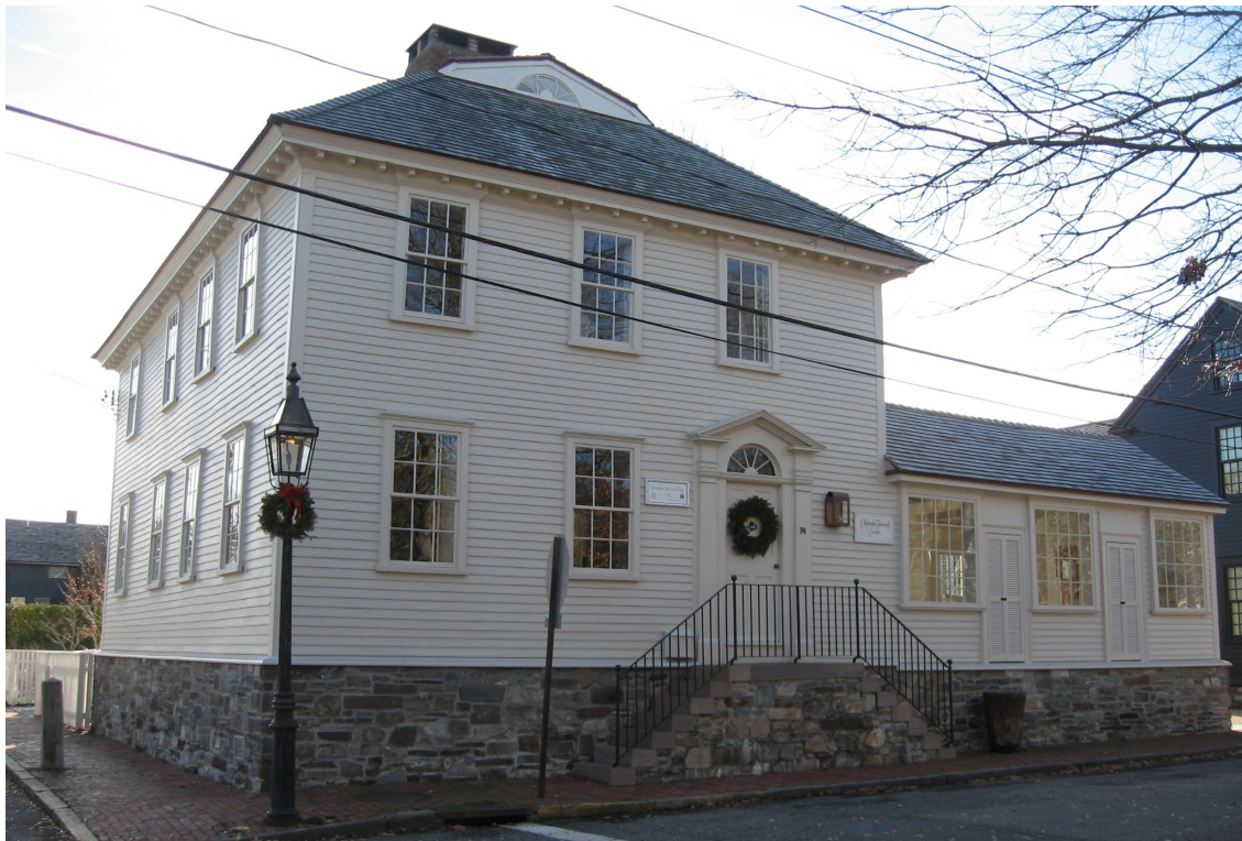
The ca. 1725 Christopher Townsend House at 74 Bridge Street is one of the first properties in Newport to be elevated using the city's elevation guidelines.
