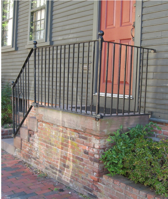
Appropriate stair designs for elevated buildings include the side/linear stair of brick construction at 11 Third Street (left) and the center/linear split wood stair of stone at 6 Bridge Street (right). Both have iron posts and railings in traditional Newport designs.
