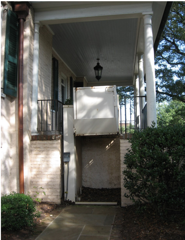
These chair lift designs provide access from a dedicated ADA parking space and required only a small section of the porches to be removed (left, Georgetown, South Carolina, right, Nantucket, Massachusetts).
