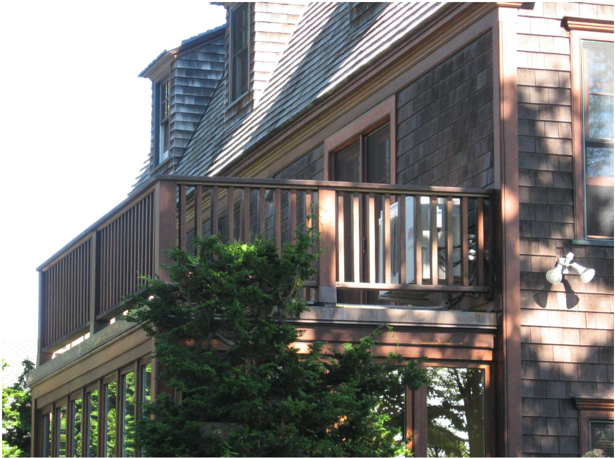
Appropriately sited and screened HVAC unit on the second floor rear porch at 52 Second Street.
