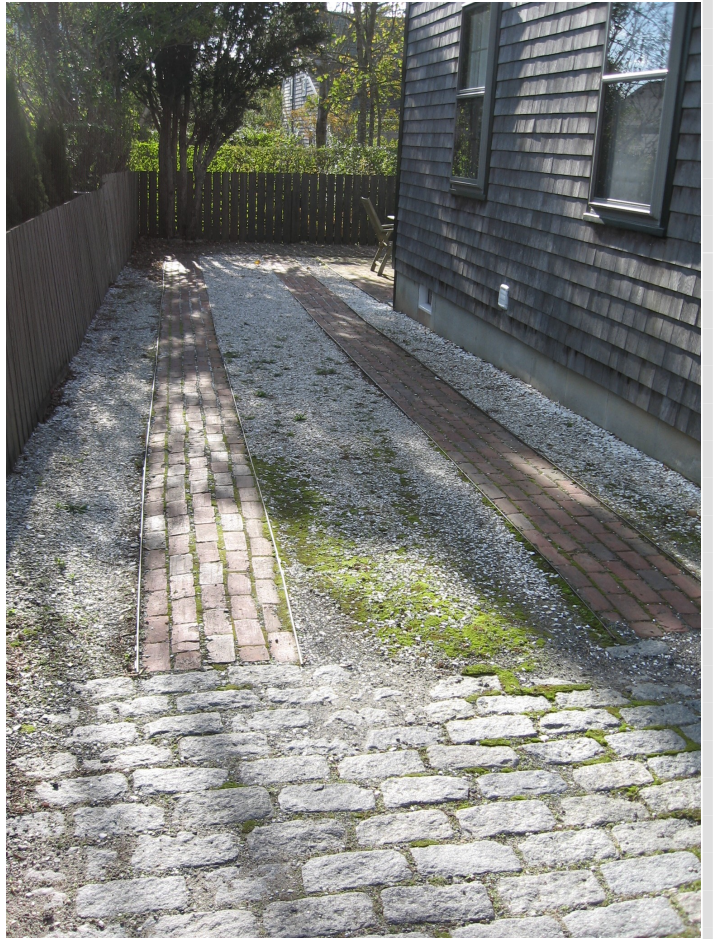
YES: Property owners are encouraged to use permeable materials for driveways such as gravel instead of hard surfaces like concrete or asphalt (left). Another approach is to only hard surface the driveway “ribbons” as shown at right (Nantucket, Massachusetts).
