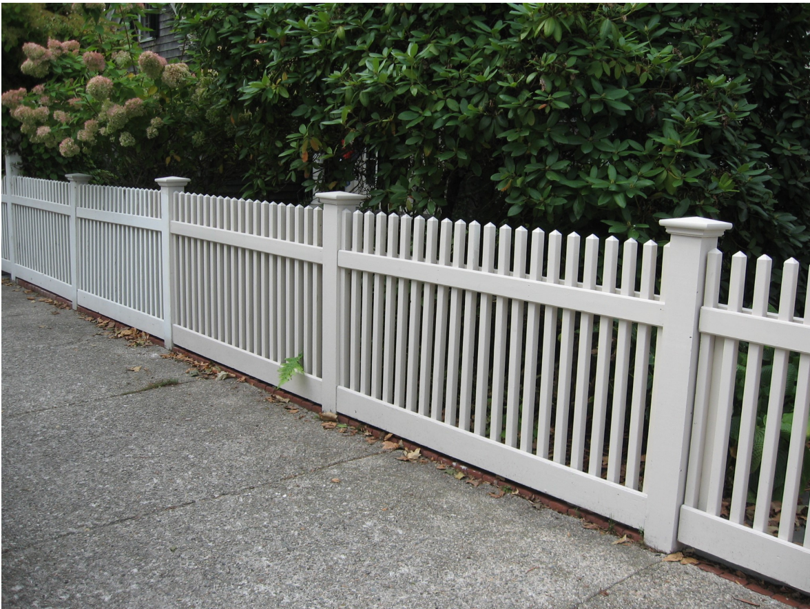
Example of an appropriate traditional fence design at 94 Washington Street.
