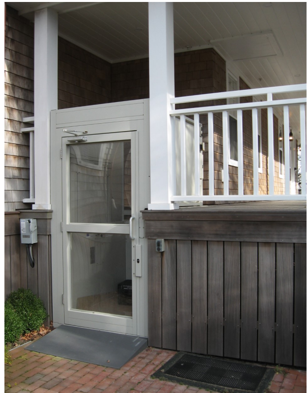
These chair lift designs provide access from a dedicated ADA parking space and required only a small section of the porches to be removed (left, Georgetown, South Carolina, right, Nantucket, Massachusetts).
