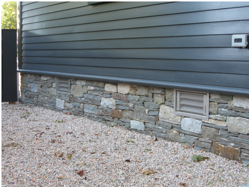
These flood vents are appropriately sited on the side elevation of the dwelling at 78 Bridge Street.
